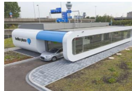
Left: A drive through battery swapping facility
